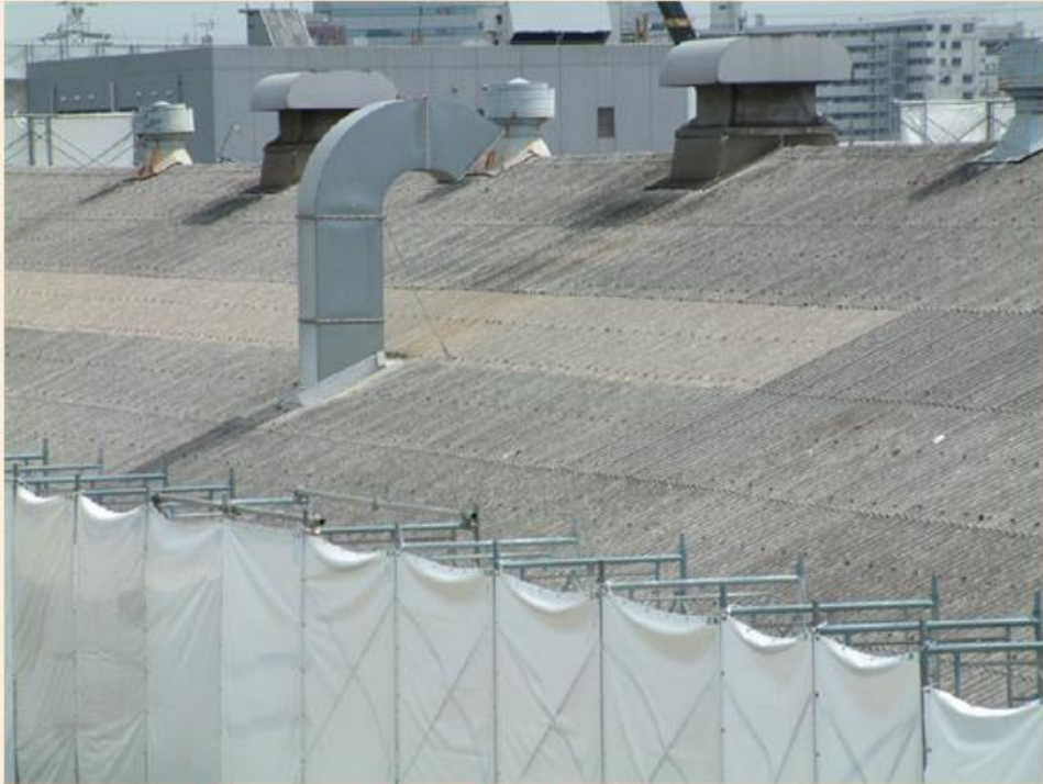
The roof contains asbestos
